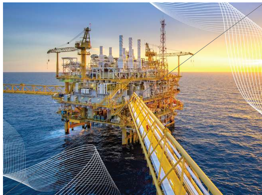
Do not use more than one set of energy lines on the same scene.
